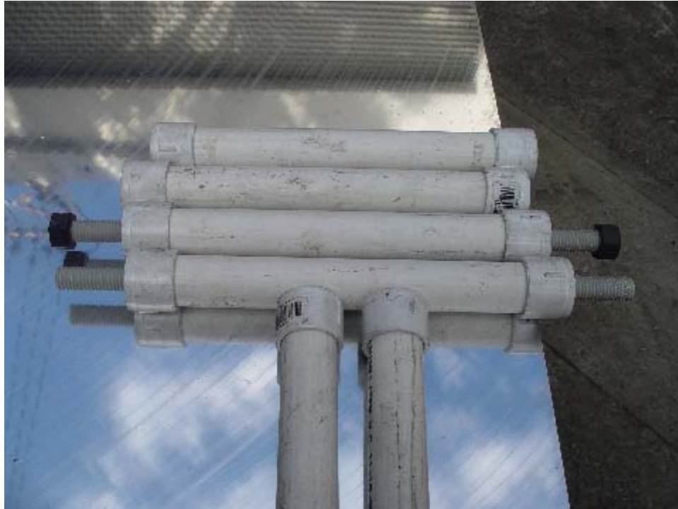
Fiberglass threaded rod now inserted into spacer bars
