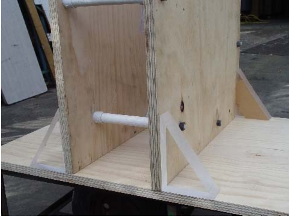
Plexiglass wedges cut and doubled up using Plexiglass adhesive.
