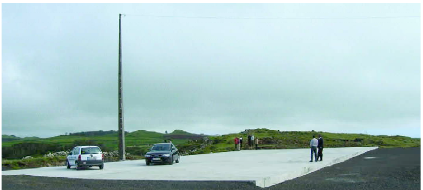
The site for the new ground station in 2006, with concrete platform, access road, power supply and lightning protection
