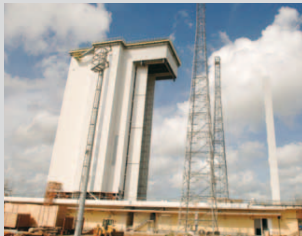
The Vega Mobile Gantry at Kourou (ESA/CNES/Arianespace)
