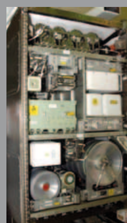
Water Recovery System 1
