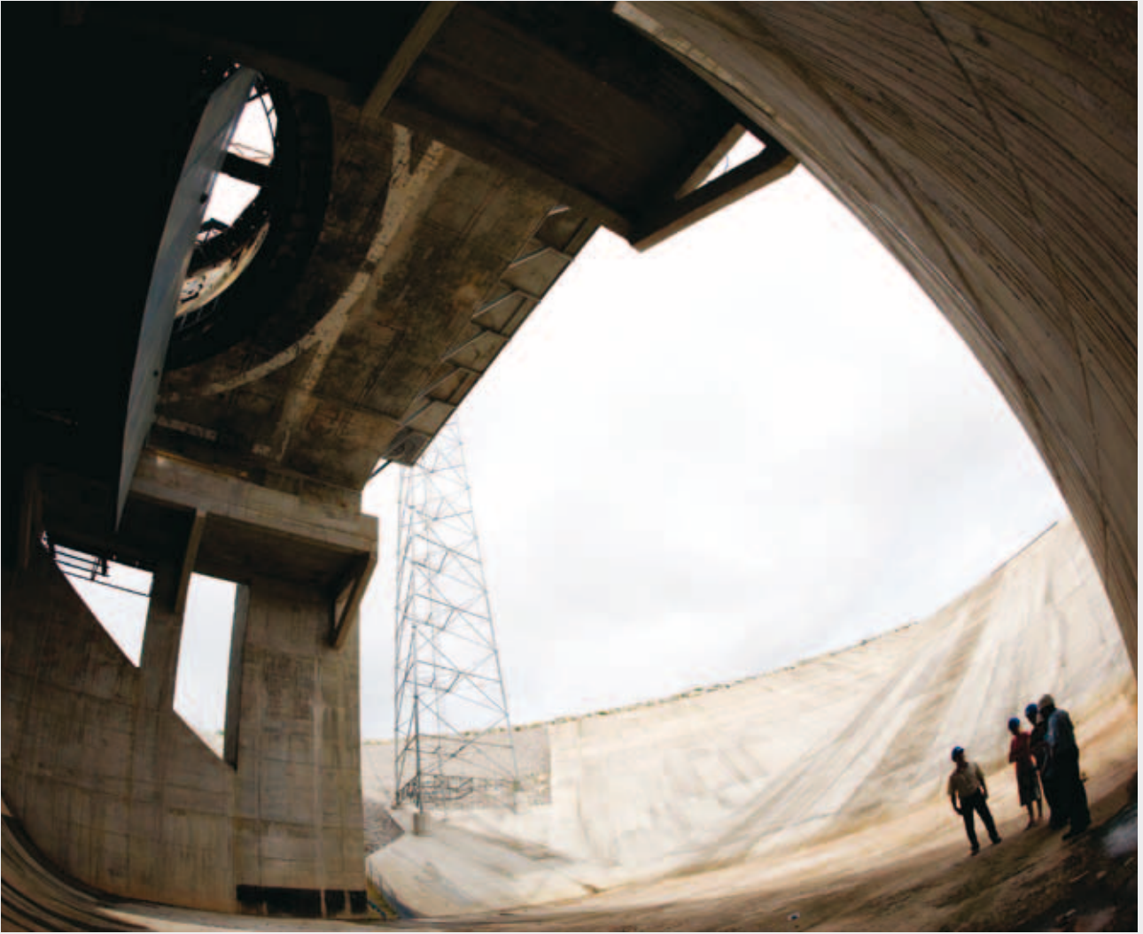
View from the flame trench underneath the Soyuz at CSG launch pad
