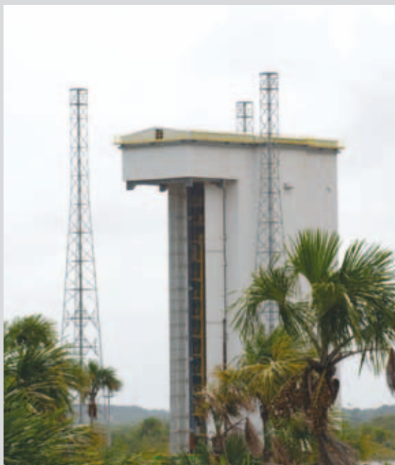
The Vega Mobile Gantry at Kourou (ESA/CNES/Arianespace)
