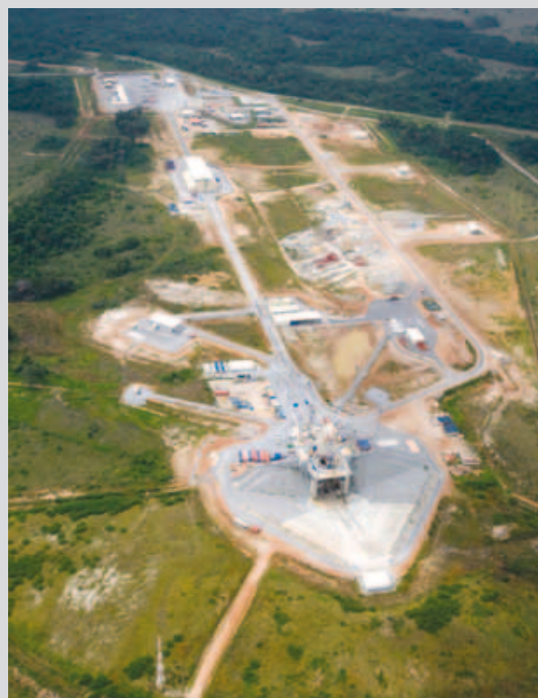
Aerial view of the Soyuz at CSG launch pad taking shape
