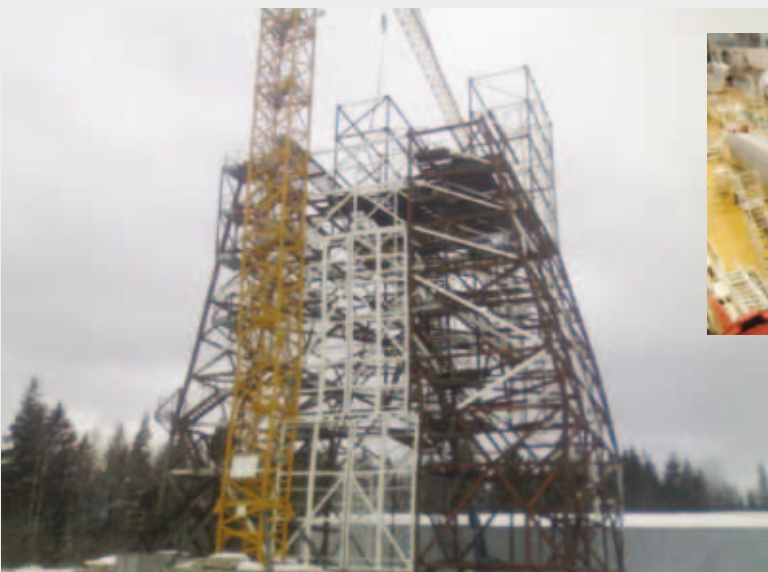
Soyuz Mobile Gantry assembly in Sergiev Posad, Russia
