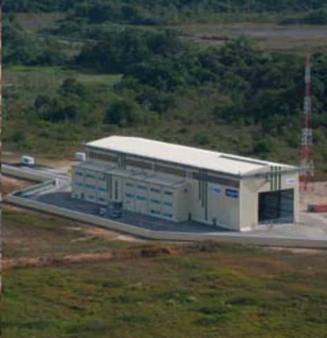
↑ Soyuz MIK launcher assembly and testing building
