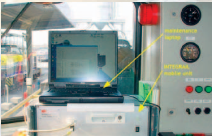
The INTEGRAIL unit installed in a locomotive for test purposes (Courtesy of Bombardier GmbH)
