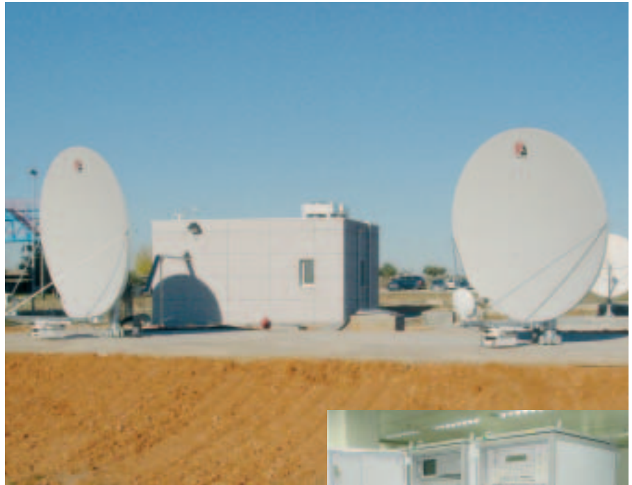
The AmerHis in-orbit testing (IOT) station, antenna and shelter and (right) the ground-support equipment used for IOT
