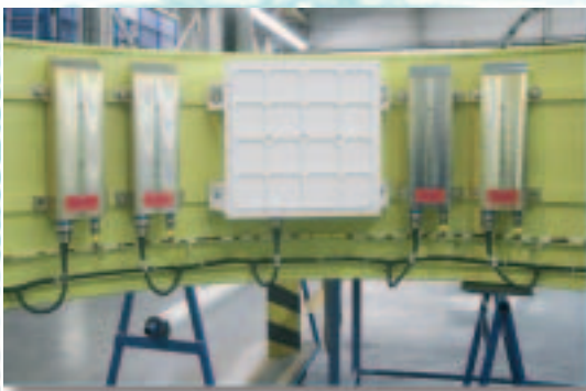
The completed interstage-0/1, developed by SABCA (B). The large box is the Control & Power Distribution Unit (SABCA, B), flanked by four Li-ion batteries (SAFT, F). This model will soon complete qualification mechanical tests.
