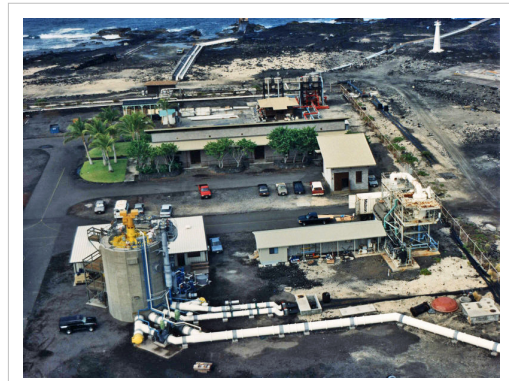
View of a land based OTEC facility at Keahole Point on the Kona coast of Hawaii (United States Department of Energy)
