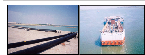
Left: Pipes used for OTEC. Right: Floating OTEC plant constructed in India in 2000
